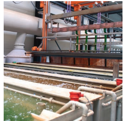
DURALLOY®-Anlage in Villingen-Schwenningen
